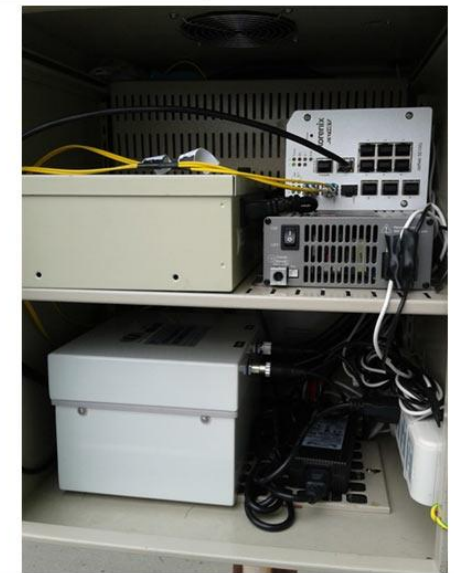
4. Street lamps DC UPS power system and 12VDC to 110VAC converter & optical transponder install images, total install 14 Unit Street lamps DC UPS for Point 1 ~ Point 16
