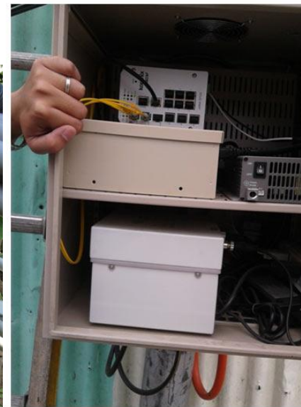
4. Street lamps DC UPS power system and 12VDC to 110VAC converter & optical transponder install images, total install 14 Unit Street lamps DC UPS for Point 1 ~ Point 16
